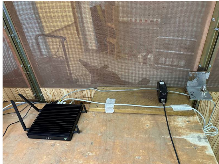
Photograph 9.2.1 Setup for conducted emission measurements at wired network port with current probe
